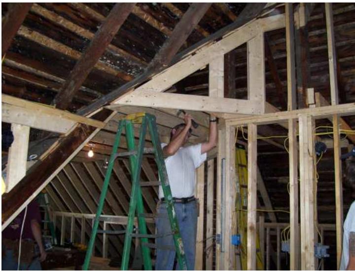
The Workcamp Crew--Third Floor Framing
